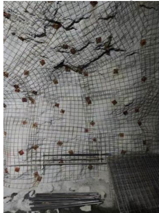
Figure 4 Bolt-mesh-shotcrete Support
